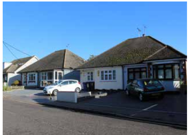
Figure 85: Twentieth century bungalows
