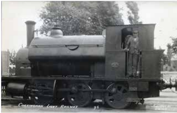
Figure 12: Corringham Light Railway (G Wood)
