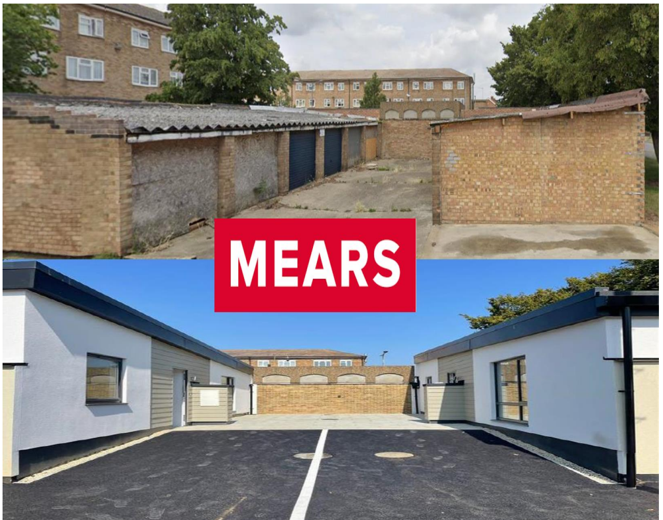
Garage area in Delargy Close – before and after
