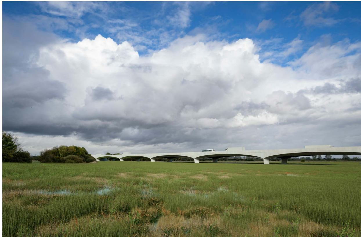
Figure 8. Artist's impression of Lower Thames Crossing Mardyke Valley Viaduct (Credit: National Highways)
