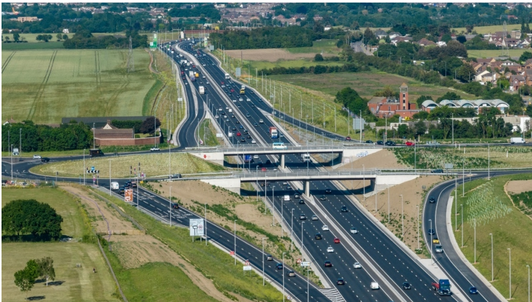
Image 1 Completed and fully operational A13 Dualling project
